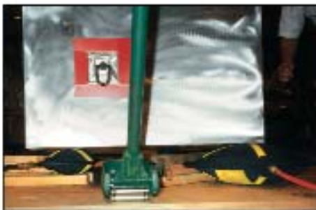
Raise loads to place industrial rollers.
