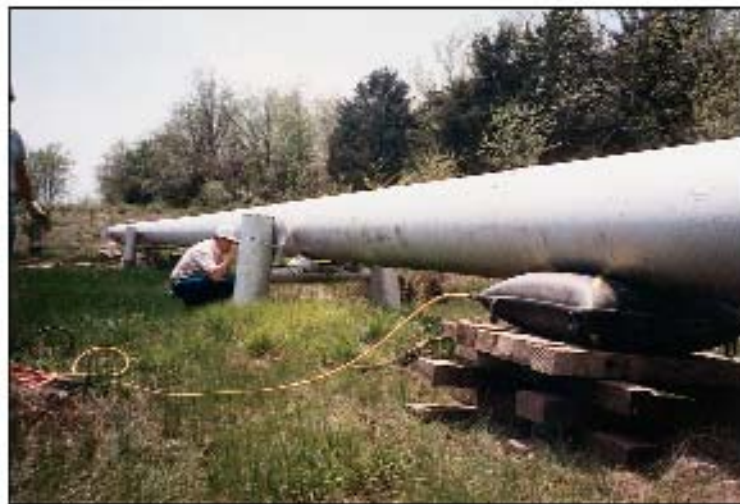
Lift and level pipelines not accessible to heavy equipment.
